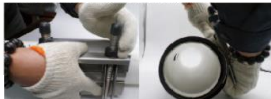
Step3 Assemble the clamp around the pipe by bringing the lock plate over the alignment lugs and hand tightening the nuts to hold it in place.
