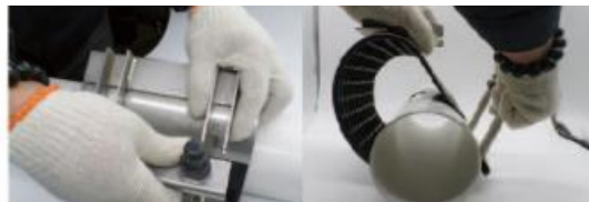
Step2 Wrap the clamp around the pipe, take note to make the overlap of the rubber away from the leak point
