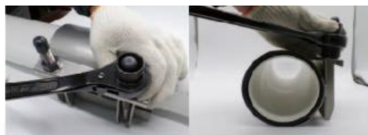
Step4 Use a tension wrench to sequentially tighten the studs to the recommended tension specified on the clamp.
